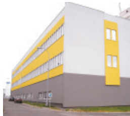
▲ Environmentally conscious plant adopting insulation board as material of its external wall
