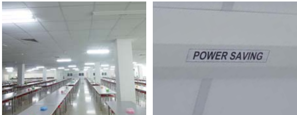
A room with a reduced number of lamps but of necessary brightness
