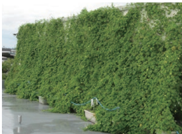
Green curtain on the wall of the plant's administrative building
