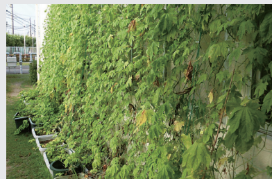
Green curtain on the wall of the plant's administrative building
