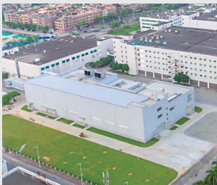
The new plant
