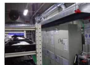
Newly installed VOC collection equipment
